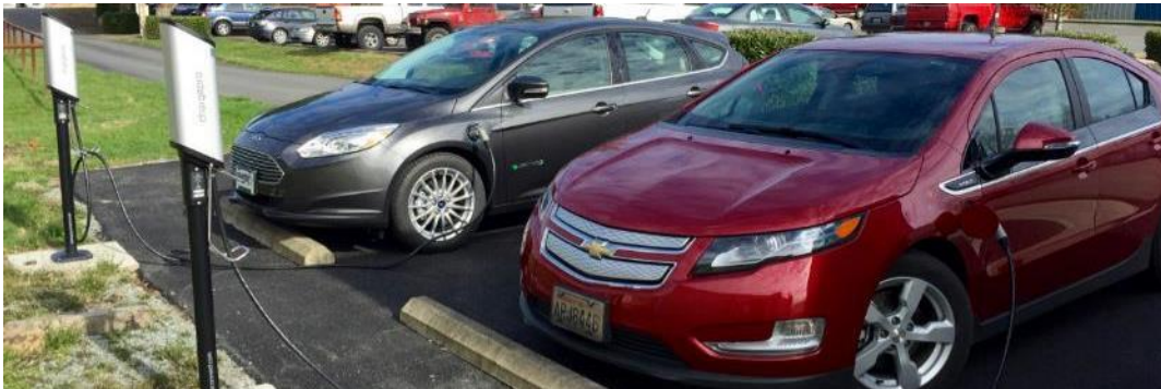
NW WA Electrical JATC EVSE Lab - Photo courtesy of Ryan Bradt
